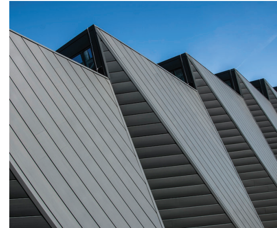
Figure 3: Materials Source: Dezeen, Switchgear Station, C.-F. Møller
