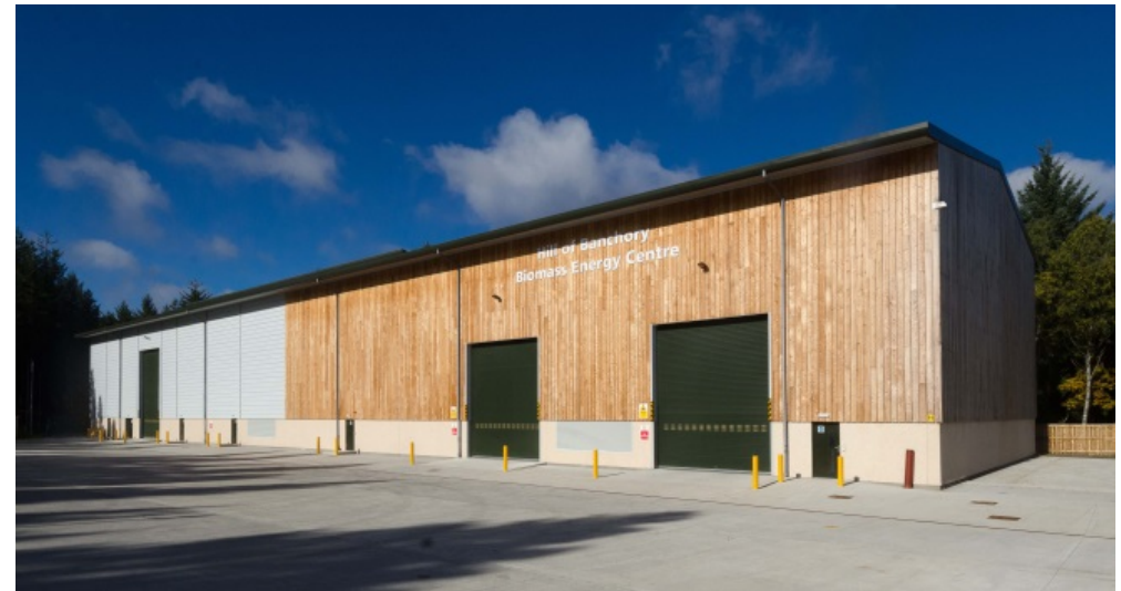
Figure 4 Biomass centre with wooden cladding
